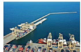
Marine Piling, Ports & Harbour
