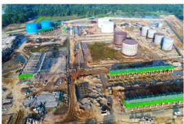
Vibro Stone Column, Oil & Gas
