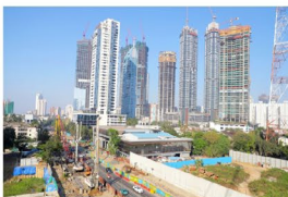
Secant Piling, Transportation-Metro
