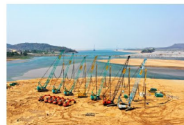
Vibro Compaction, Hydro & Irrigation
