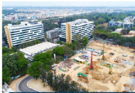
Piling, Industrial Buildings
